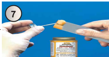
Solvent Cement Application
