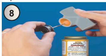
Solvent Cement Application
