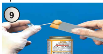
Solvent Cement Application
